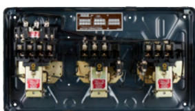
Interior View of MK1 SASD
