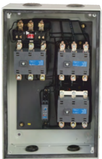
Interior View of ML FASD
